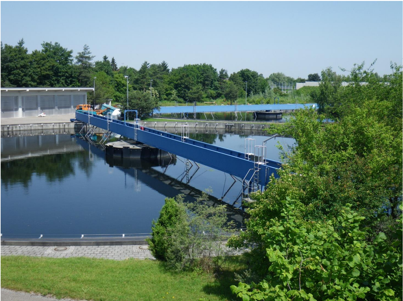
Augsburg municipal sewage treatment plant (source: City of Augsburg)
